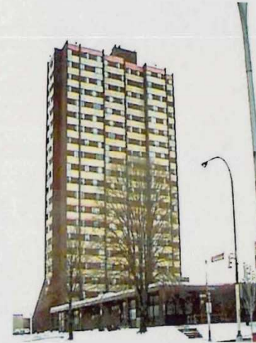
Penn Circle Towers
